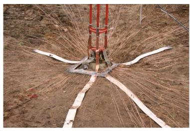
bad ground system can lead to many difficulties. By ensuring a good ground system we head off problems further down the line in our station systems. A poor ground system will limit our stations. They will never live up to their highest potential.
